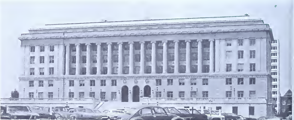
South elevation of the North Office Building.
